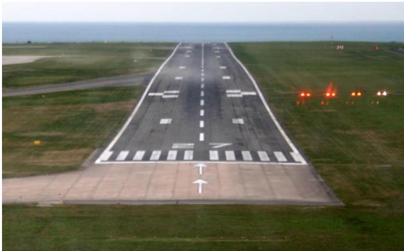
**Visual Approach Slope Indicator** - The VASI consists of a red bar of lights, and a set of white lights in front of them. At the correct slope, the white lights are aligned with the red bar. At the SLF, the VASI is located about 670 meters behind the runway threshold.
